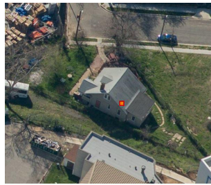
EXISTING VIEW FROM SOUTH
